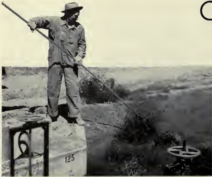
CLEANING WEEDS FROM A TURN-OUT.—William Amoureux, ditchrider in the Winchester water section, uses a long-handled weed fork. Photo by F. B. Pomeroy, Region 1 photographer.
